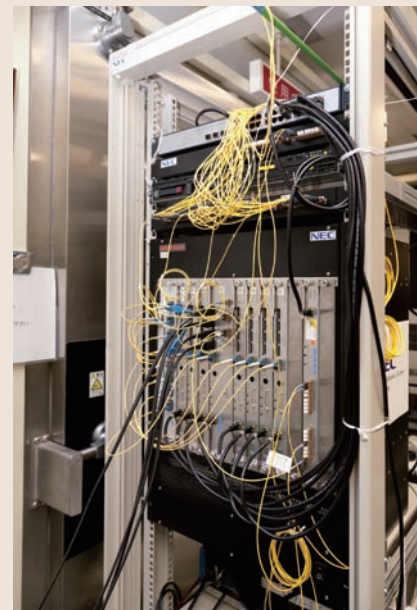
Figure 5 ● Monitoring Equipment of Quantum Cryptography Network For general market penetration, its size reduction is required.
